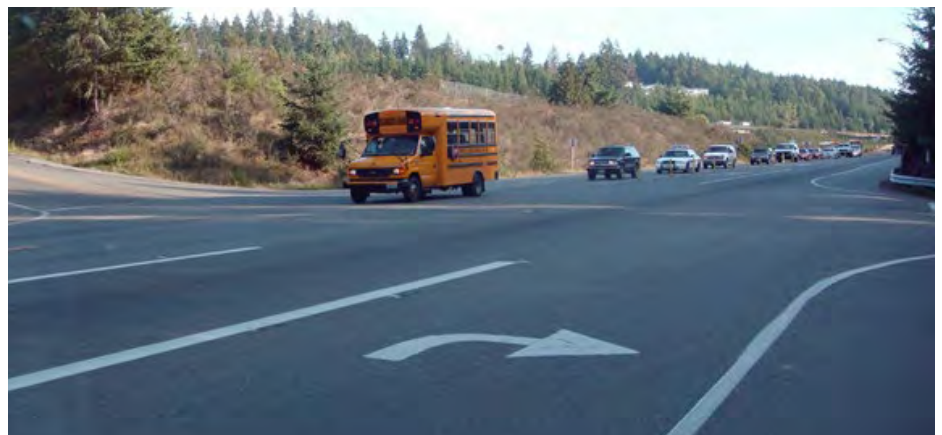
Example of a right-turn lane.
