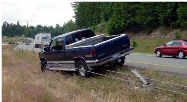
Median cable barrier prevents a potential head-on crash.
