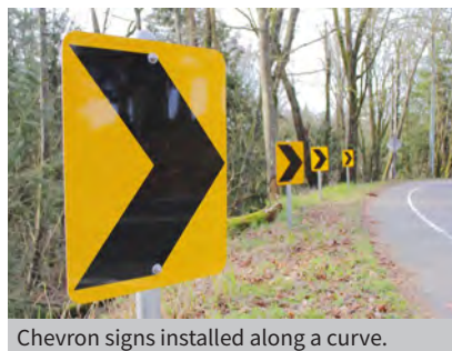
Chevron signs installed along a curve.
