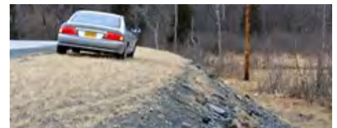
Shoulder is provided along roadway curve.
